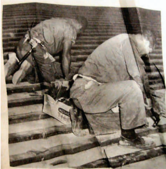
CARPENTERS LAYING SLEEPERS FOR THE GYMNASIUM FLOOR OF NEW SCHOOL.
